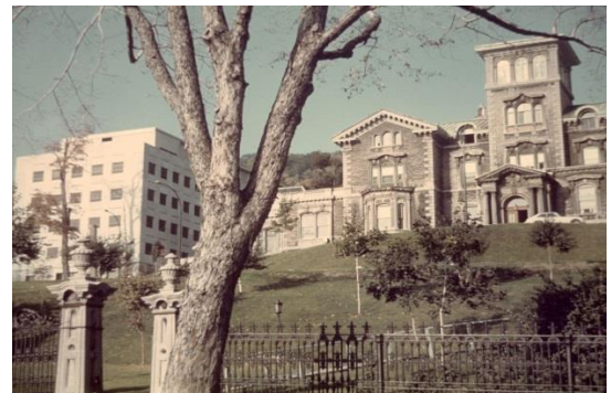
Ravenscrag (1893), opened as the Allan Memorial Institute for Royal Victoria Hospital and McGill Psychiatry Dept., 1944
