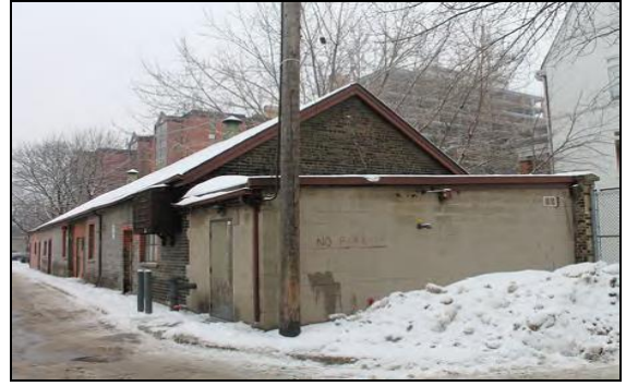
Concrete block addition on west end of the East Workshop
