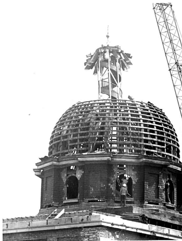
During demolition in 1976 of the original Queen Street asylum structure, built 1846-50, a crane extracted the “flying staircase” for preservation as an artifact. Photo print: CAMH Archives, Queen Street fonds, 32-21.
