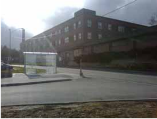
Nicholls Building, Peterborough
